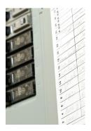
• Label all circuit breakers and fuse boxes clearly. Each switch should be labelled to indicate which outlet or appliance it is for.
